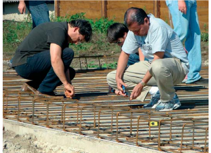
Citi participation in Habitat for Humanity House Building Volunteer Program in Hajdúböszörmény
